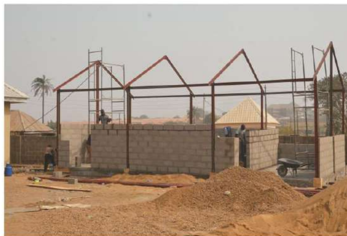
The site for the installation of the grinding machine under construction.
